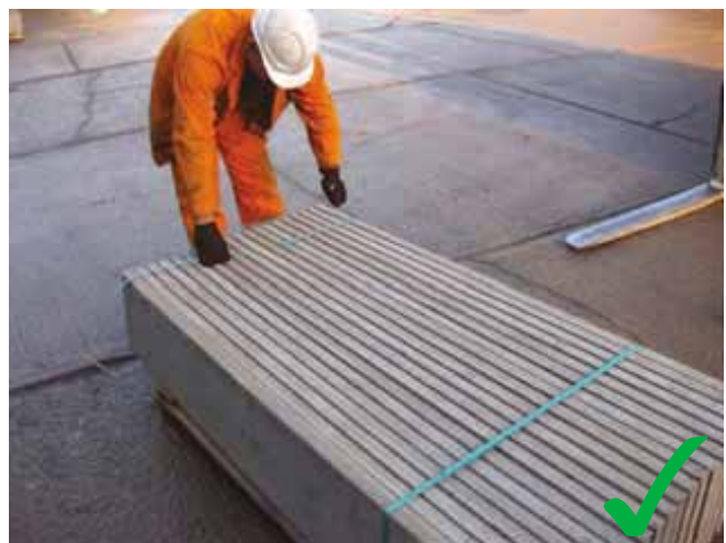
Products MUST NOT be taken out of packs using the forklift, they will damage the unit. Care and attention must be paid when opening gravel boards. Always leave the band holding just part of the pack, this will prevent the whole pack collapsing when the pack is opened (as shown above).
