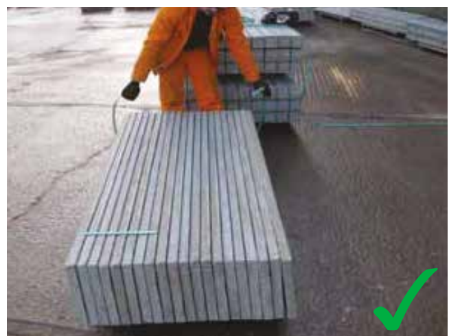
Products MUST NOT be stacked unevenly. When both main bands are removed from gravel board packs the pack should remain standing when the part band is left. However, you will need to support the front board initially when opening fully. (as shown above).
